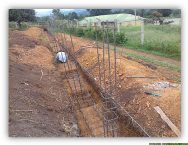
And simultaneously, a retaining wall has been and remains under construction.
