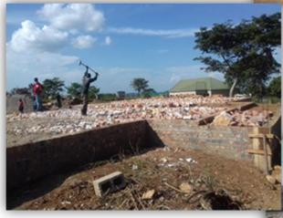
It has requires 18 trips of hard rock to level up the foundation and to make it ready for concrete slab.
